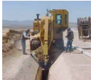
NTC Fiber Optic Network Cable Installation
