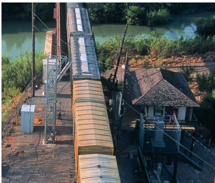
The Railroad VACIS system scans closed, moving railcars.
