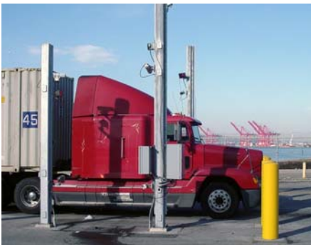
SAIC's OCR technology automatically identifies equipment at the gates and on the quay.
